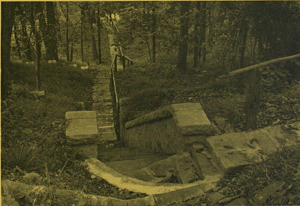
Newly laid steps from Old Hospital to Joy House cut and set by J. G. Morgan. Photographs by Gabrielle Beasley.
