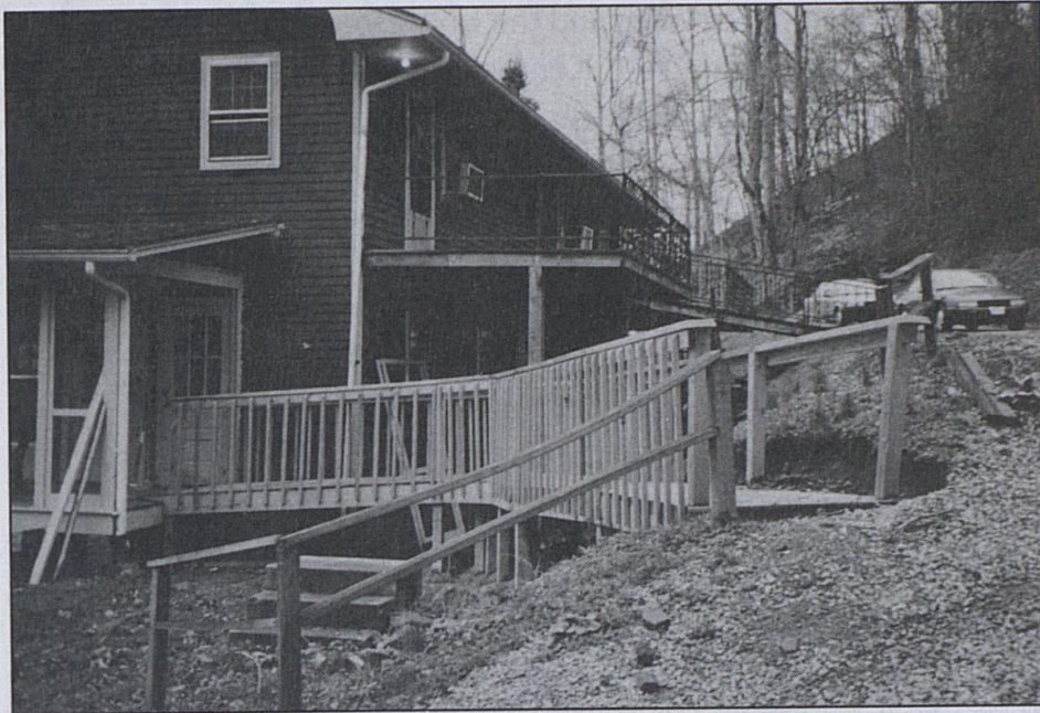
Handicapped ramp at Mardi Cottage
