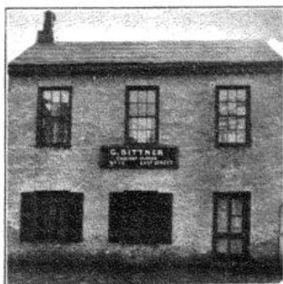
Building in which Gustav Bittner established the business which bears his name, just as it appeared sixty-nine years ago, and still part of the plant of G. Bittner's Sons.
