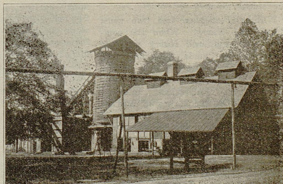
"The Firmstones being of English heredity and tradition the Longdale furnaces were built to conserve heat. The furnaces had no steel jackets, but brick walls surrounded by heavy iron bands"
