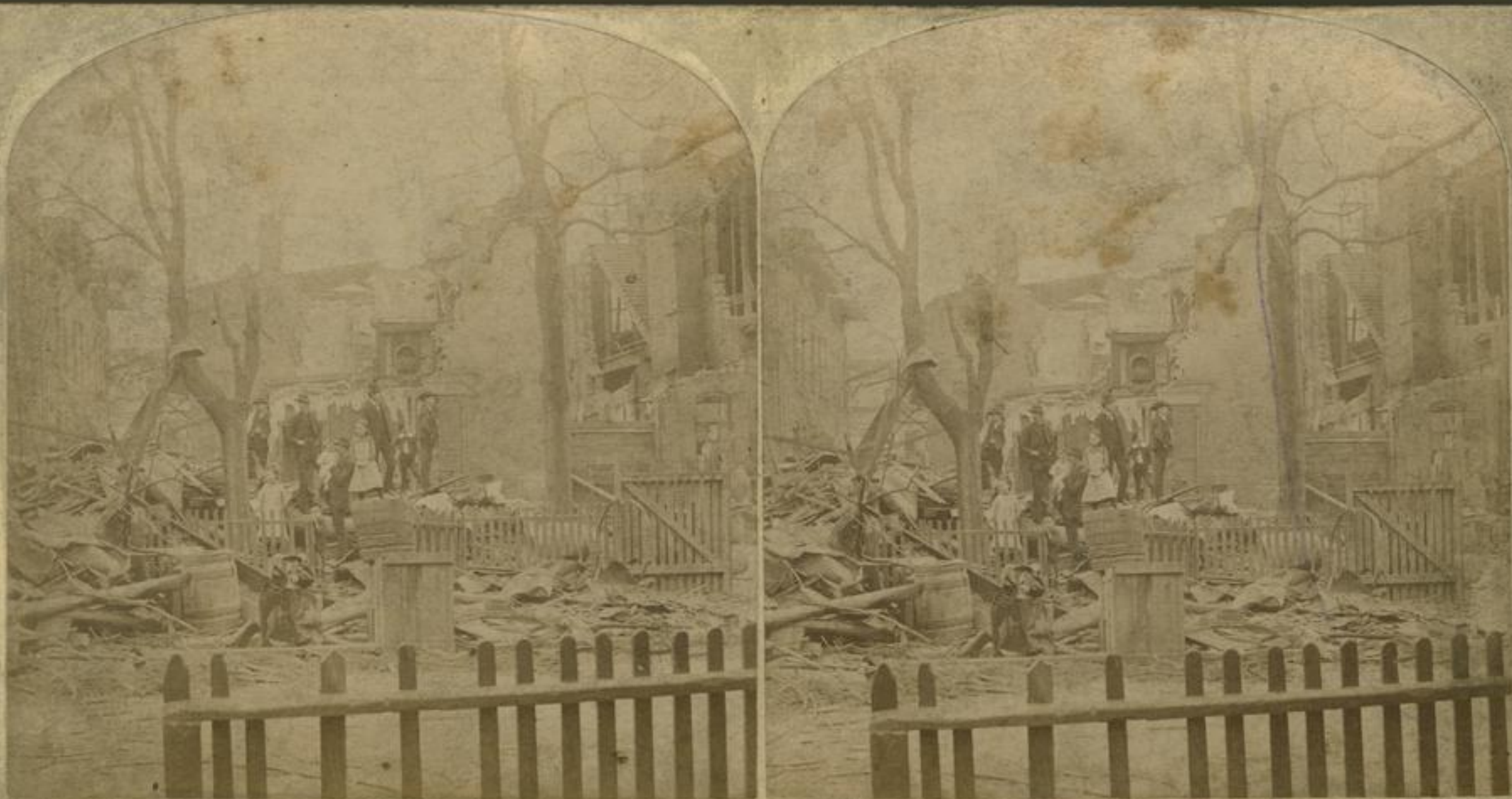
Great Tornado 1890, "Home Sweet Home" - scene of Destruction - Chapel Street.
