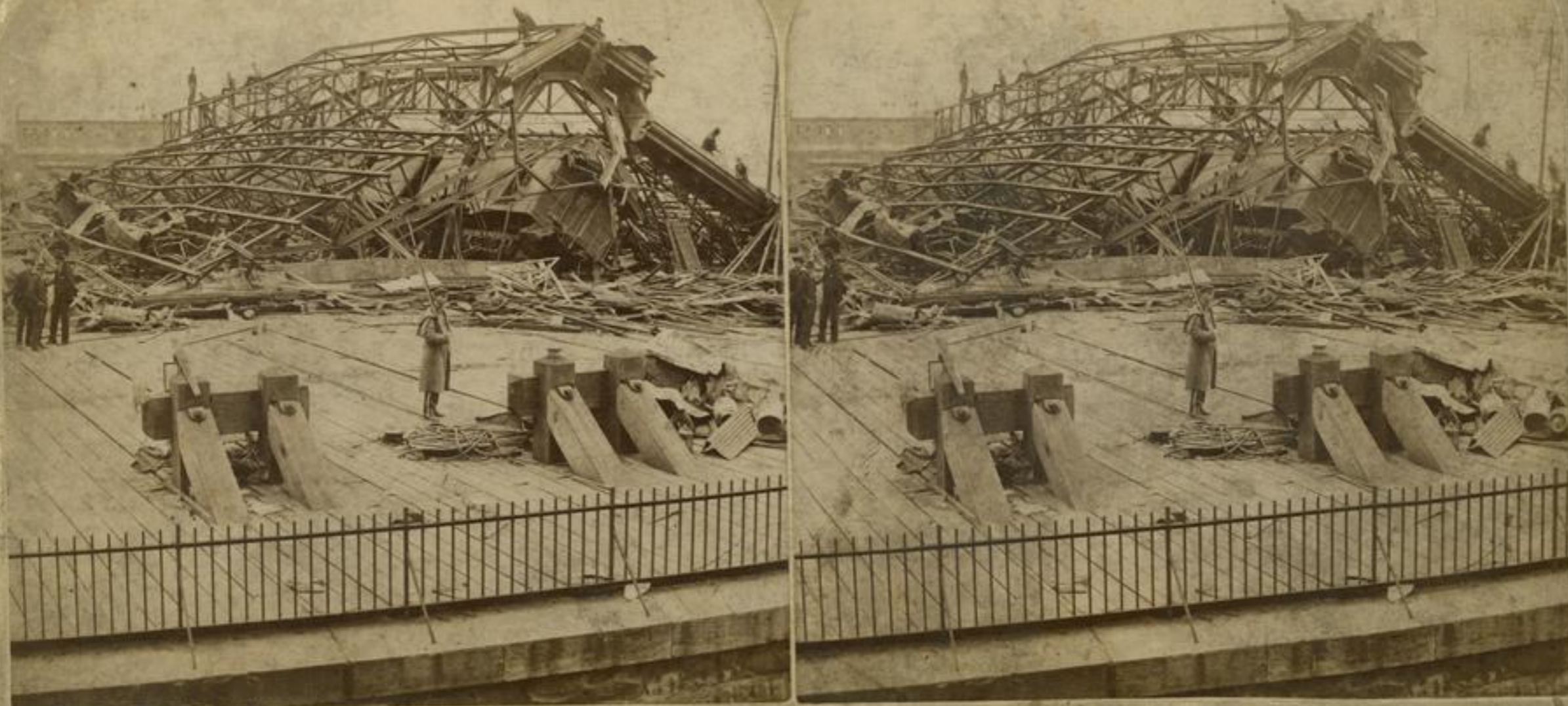
Louisville Tornado. Wreck of the Union Depot.
