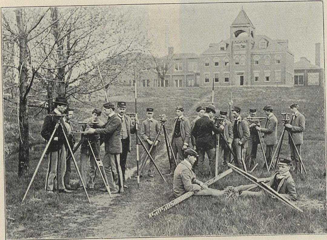
CLASS IN CIVIL ENGINEERING.
