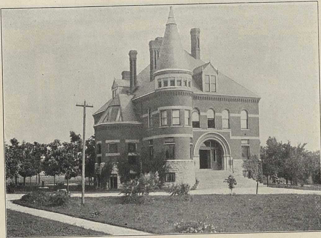
EXPERIMENT STATION BUILDING.
