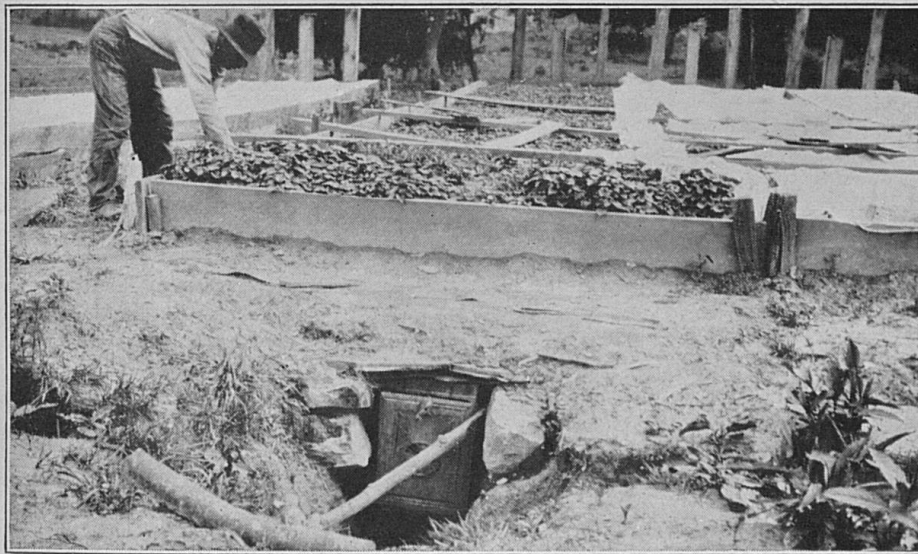
FIGURE 7. Flue-heated hotbed, showing fire-box end.
