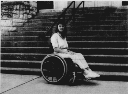
Stairs are a problem for disabled students at the Ezra J. Gillis Building, one of the few structures left on campus that has not been made handicapped accessible.
