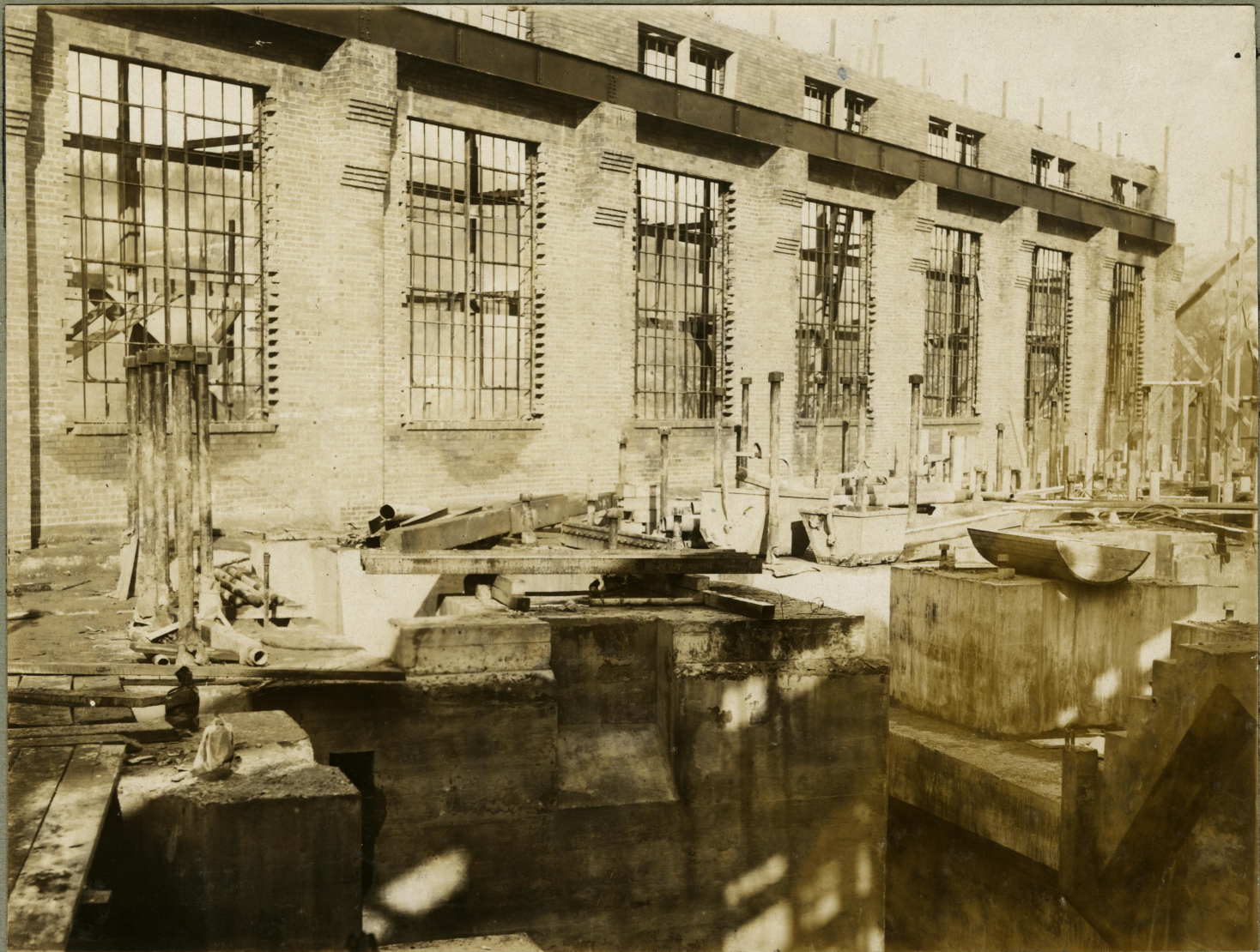
Engine Foundation ~ Dec. 12, 1914
