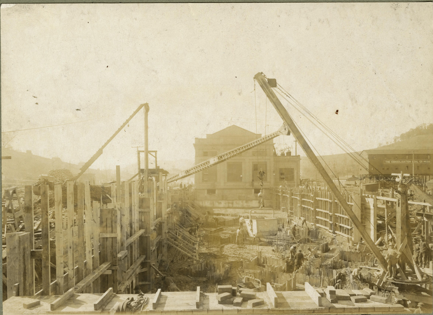
General View ~ Foundation Work
