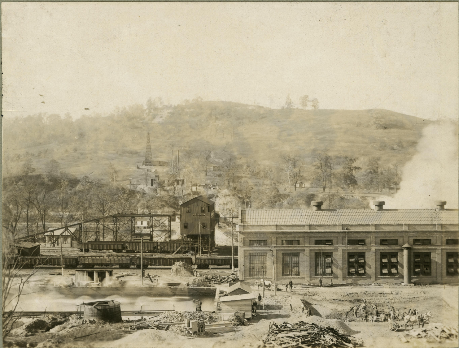
Excavation ~ Cooling Pond
