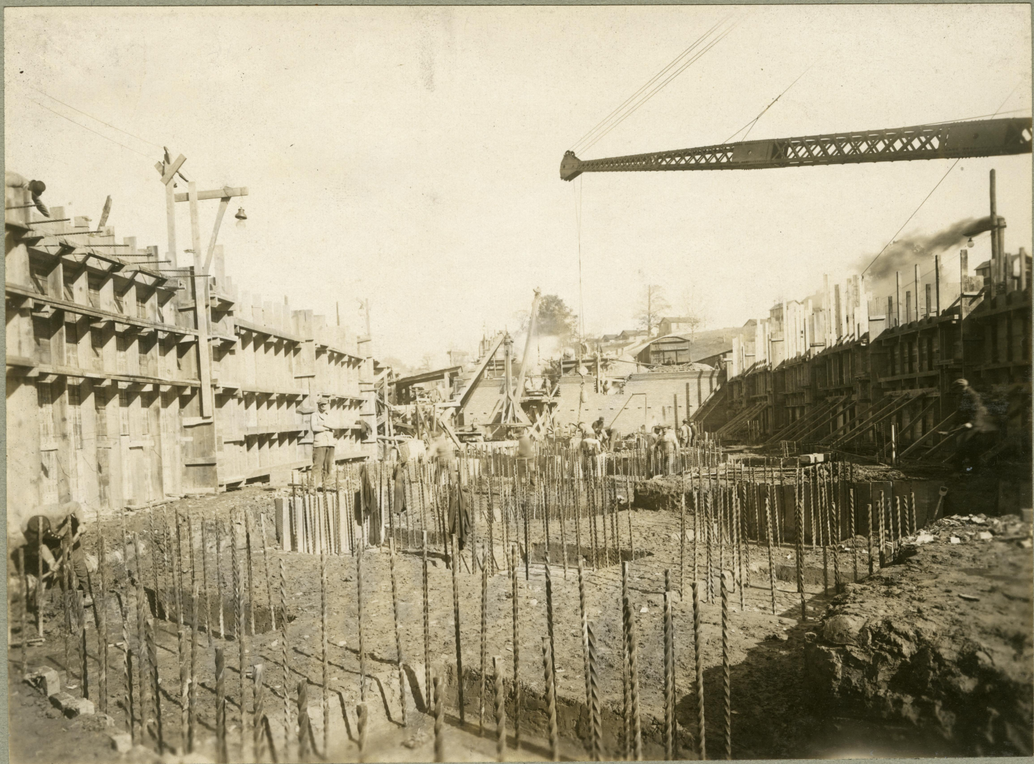
Concrete Foundation ~ Oct. 26, 1914
