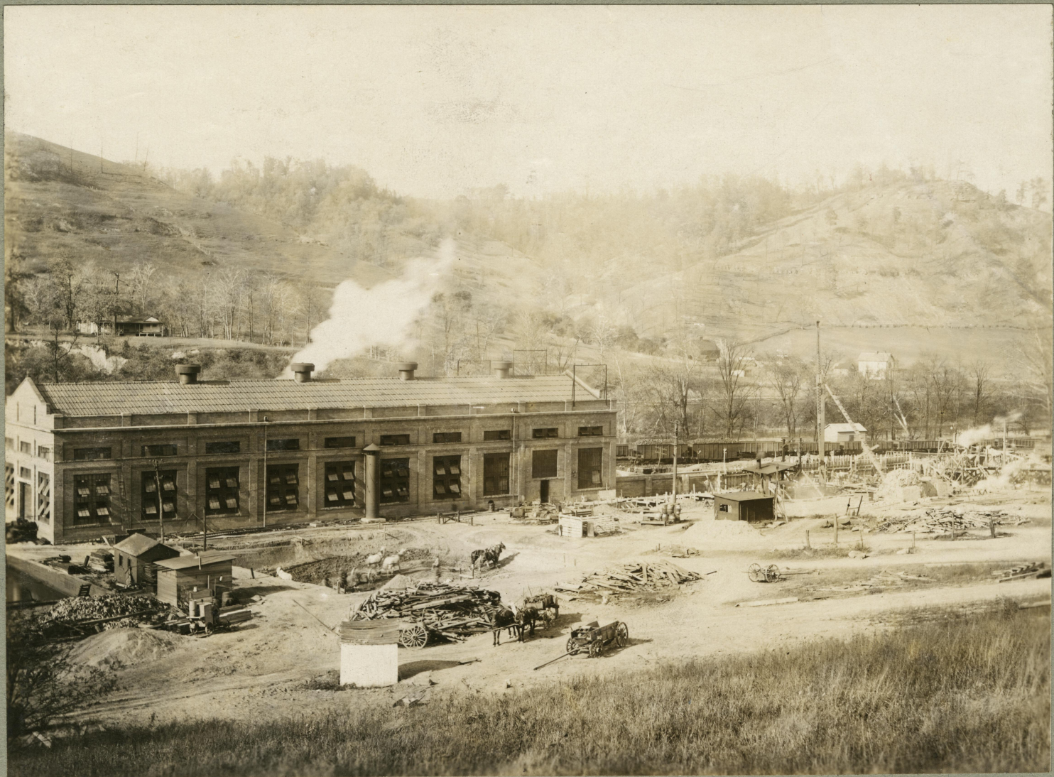
Progress on Foundation ~ Nov. 6, 1914
