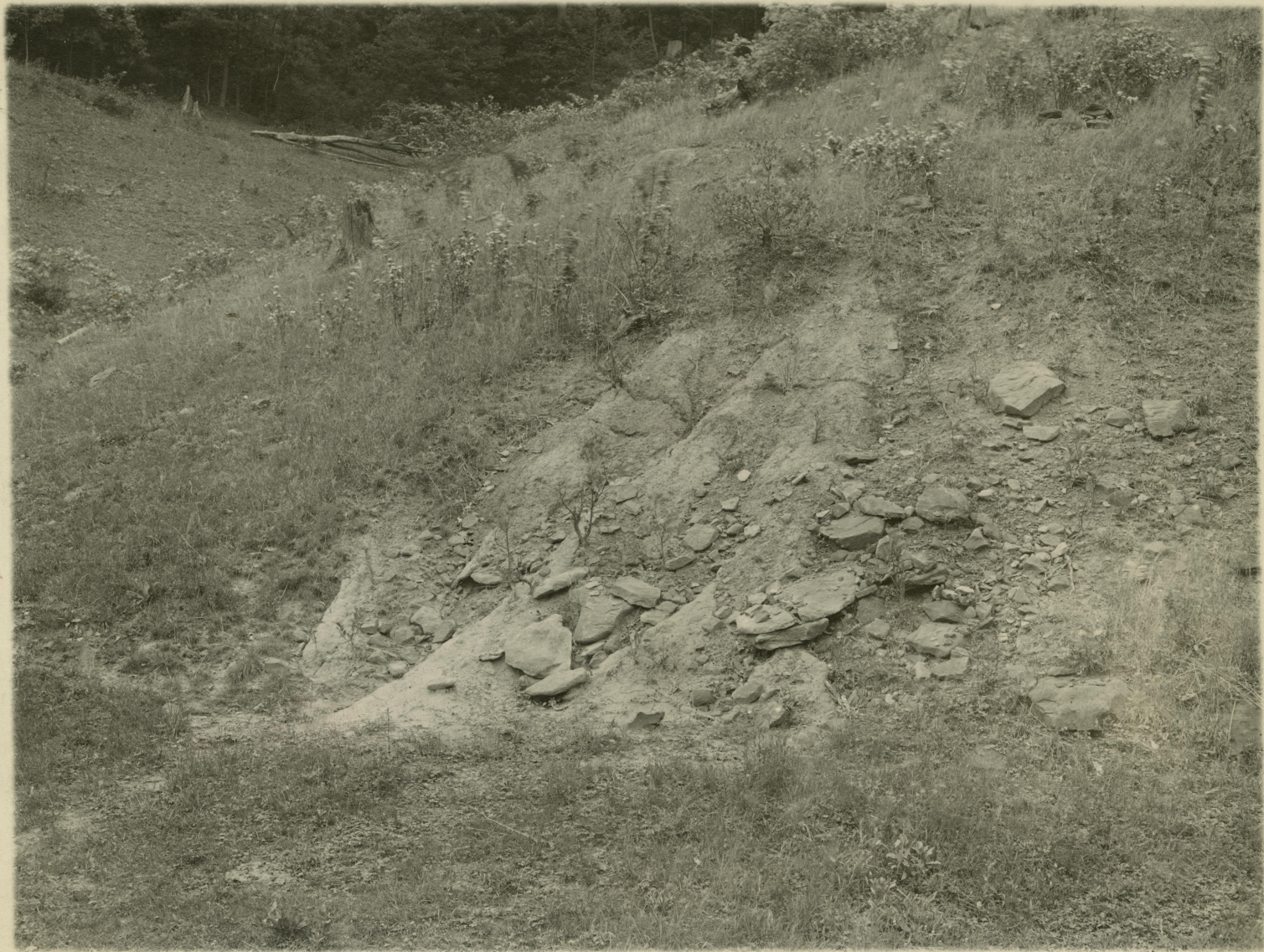
Pictures of surface breaks at Dairy, Jenkins, KY ~ May 22, 1919
