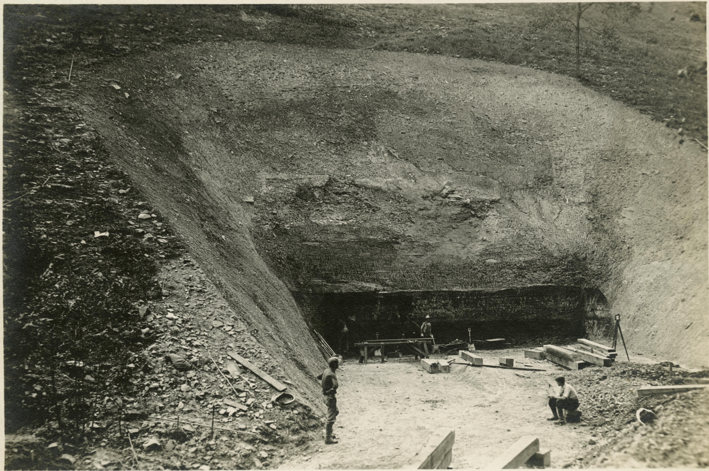
Coal faced for opening, No. 205 Mine, Sept. 22, 1911.
