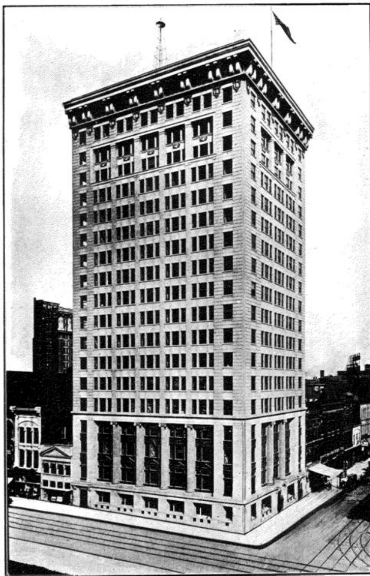
THE NEW HOME OF THE INTER-SOUTHERN LIFE INSURANCE CO. LOUISVILLE, KENTUCKY
