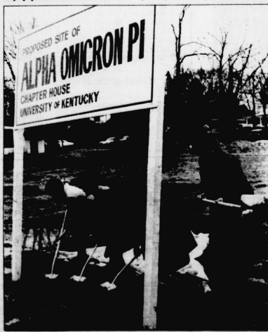
TIM SHARP/Kerbel Staff AOPi's wield shovels to break ground for their new house.
