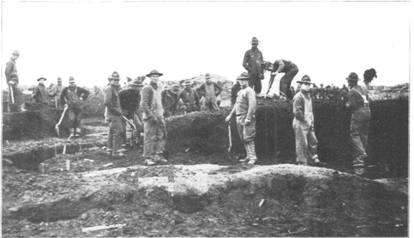
NO PLAY HERE—DIGGING TRENCHES
