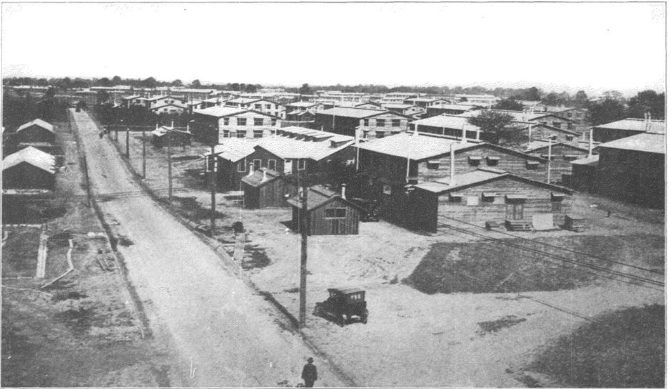
GENERAL VIEW OF CAMP TAYLOR
