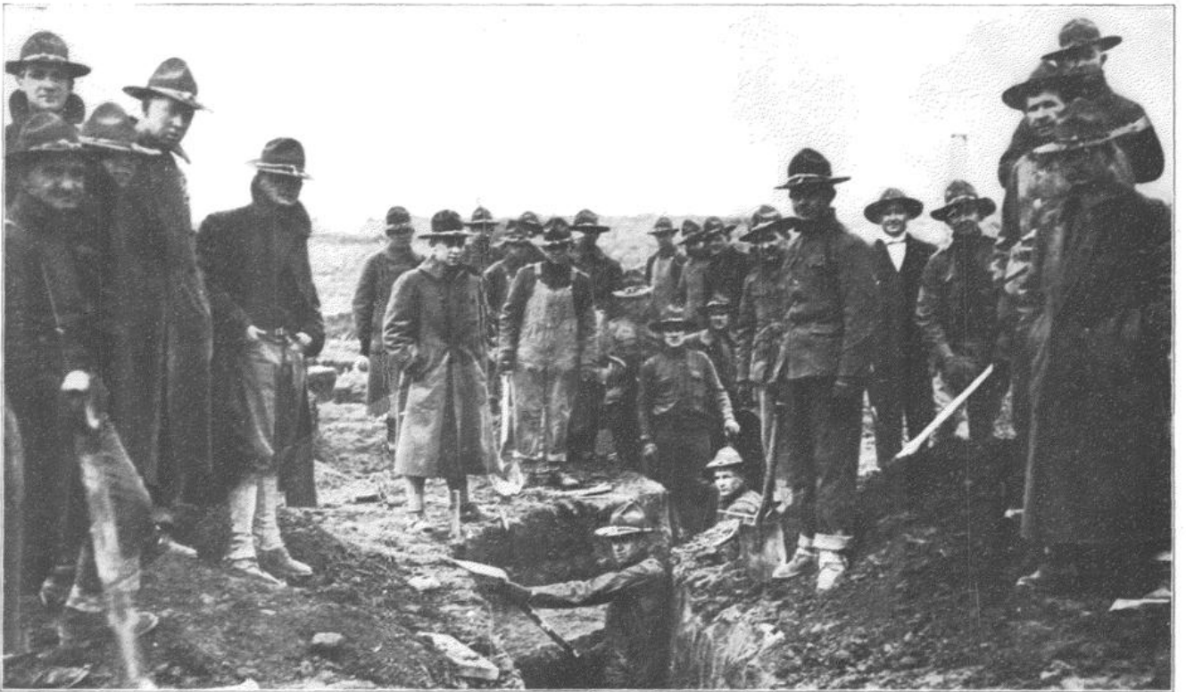
TRENCH DIGGING IN THE BIG MANEUVER FIELD
