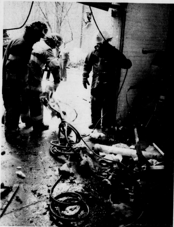
Lexington firemen examine the area where the explosion took place in the Anderson Hall Quadrangle. The explosion knocked out about 200 windows in the structure. No one was seriously injured.
