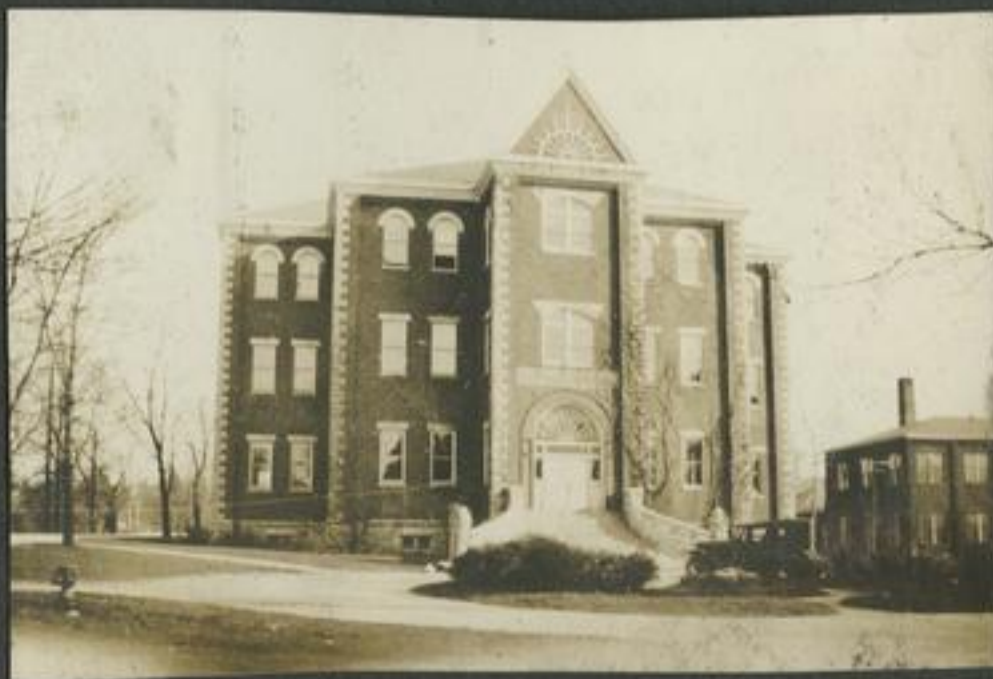
ARTS AND SCIENCE BUILDING 100
