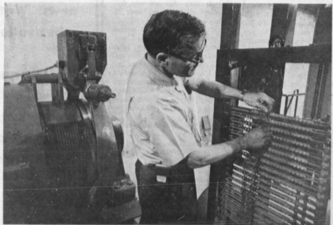
Bill Skinner, Ceder Elevator's UK maintenance man, inspects one of the relay panels which control the Office Tower elevators. To his left is the cable machinery which hoists one car up and down its shaft; five cables supply traction besides an extra safety factor.
