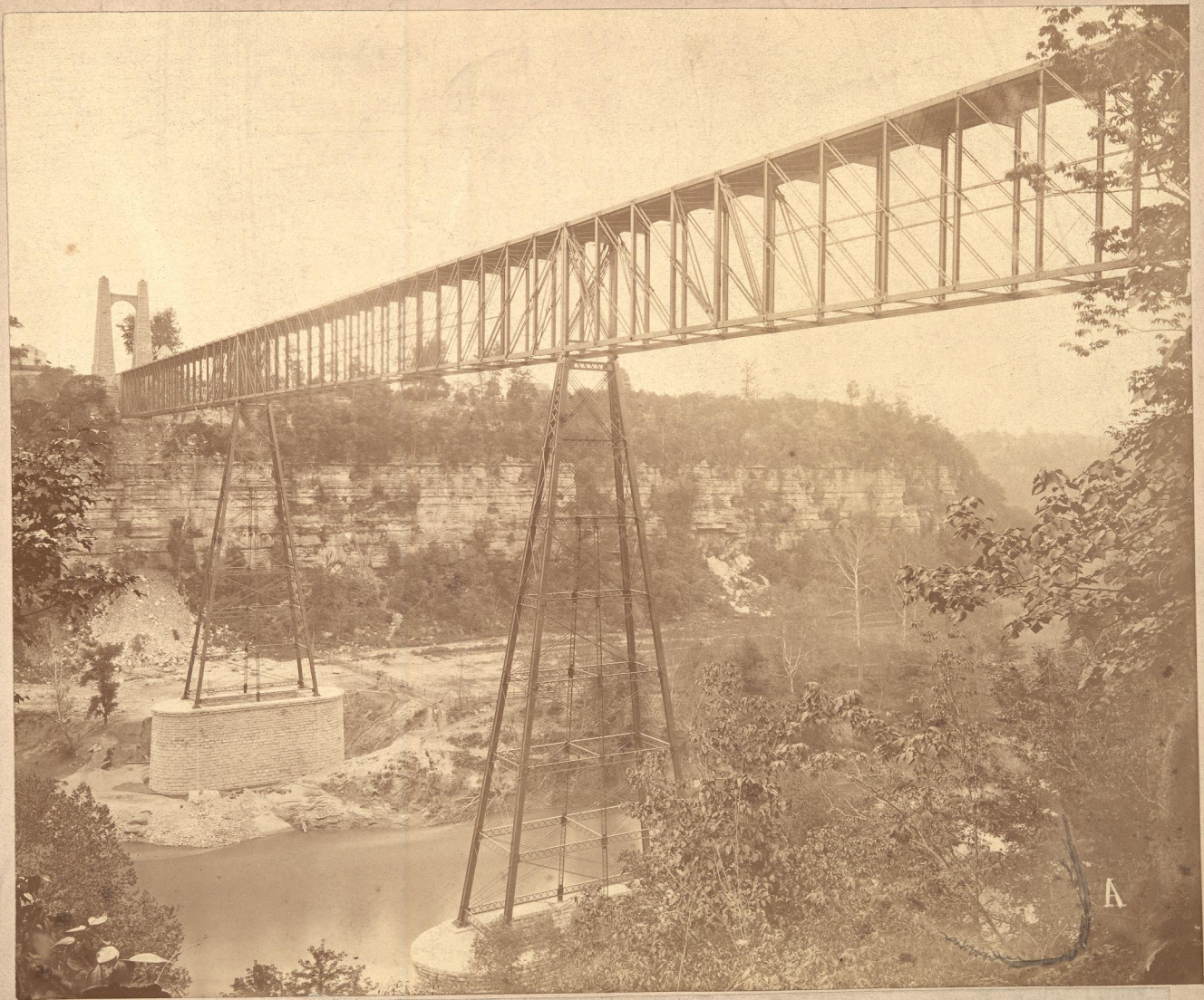
A MULLEN, Photo. LEXINGTON, KY. KENTUCKY RIVER BRIDGE--CINCINNATI SOUTHERN RAILWAY.
