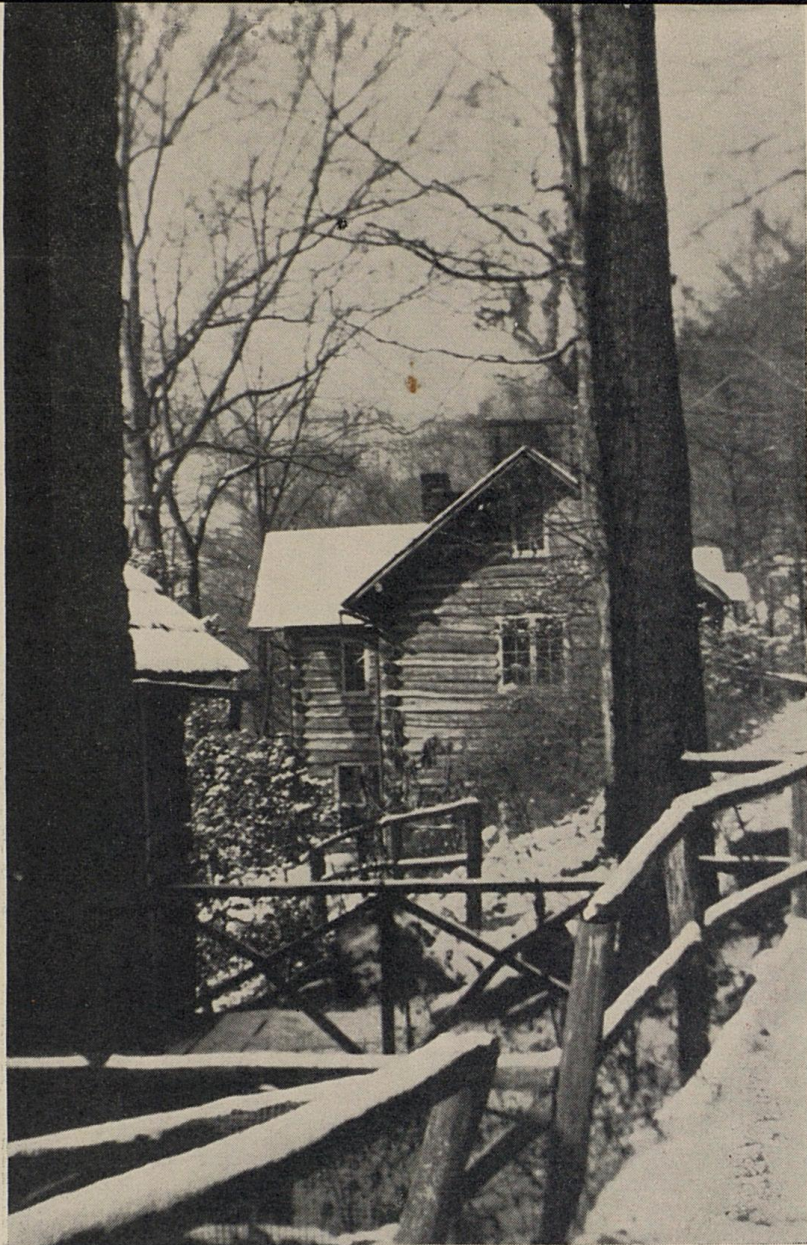
WENDOVER IN WINTER The Big Log House and a Corner of the Log Chapel
