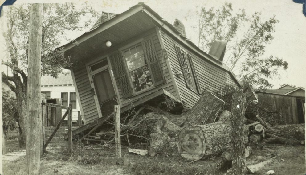
The falling tree did this to the house.
