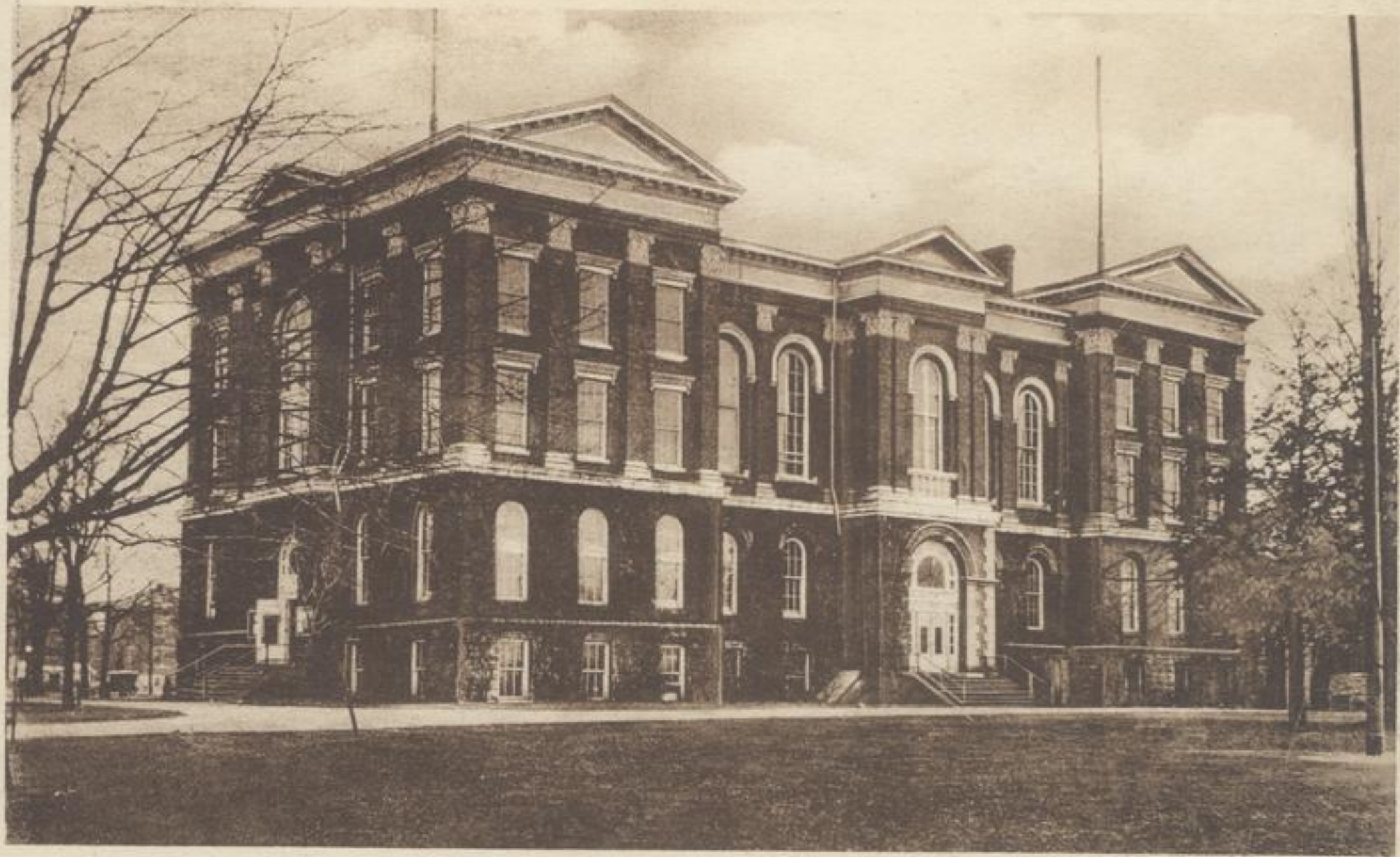
ADMINISTRATION BUILDING — UNIVERSITY OF KENTUCKY. LEXINGTON.
