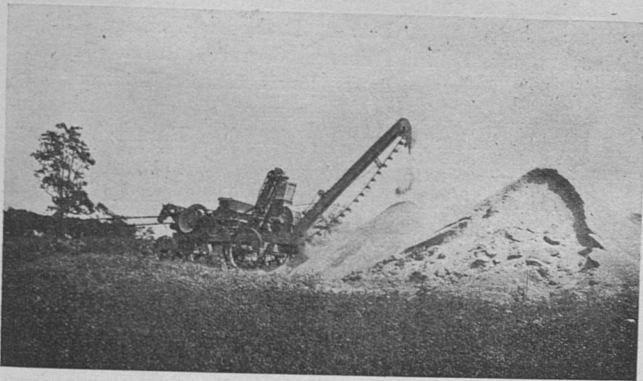
Fig. 1. Ballast Crusher and Limestone Pulver Mounted on Same Truck.
