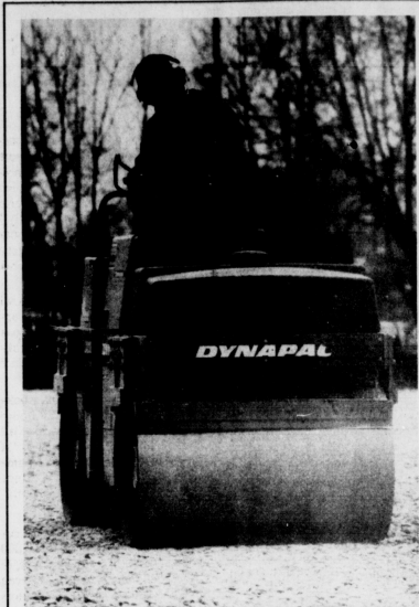
MORE PARKING: Tom McCoy of the Physical Plant Division rolls over gravel in a new parking lot behind K-Lair yesterday.
