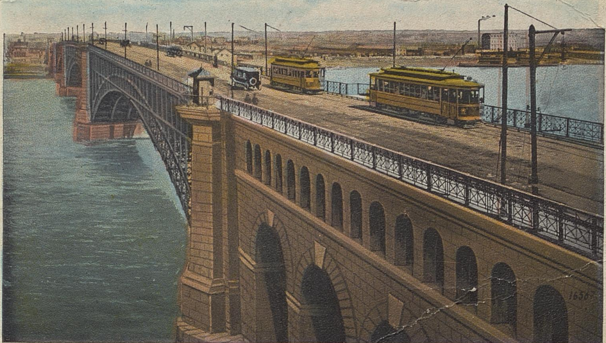
1000:—Eads Bridge, St. Louis, Mo.
