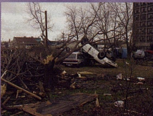
Damage reached epic proportions as tornadoes cut a wide swath through much of Western Kentucky.
