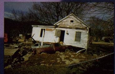
The 1997 flood ravaged any number of cities and counties in Kentucky, causing hundreds to flee their homes.
