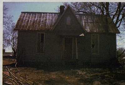
A flood-ravaged home
