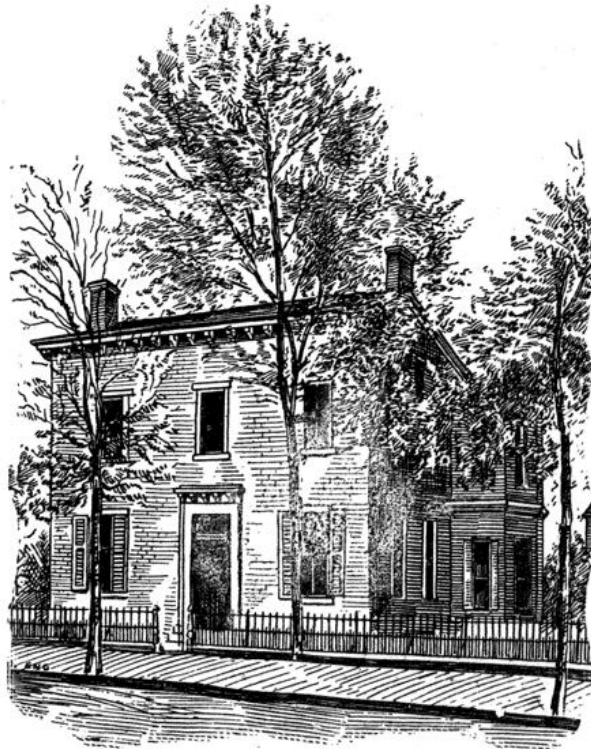
TORN AWAY IN 1895
