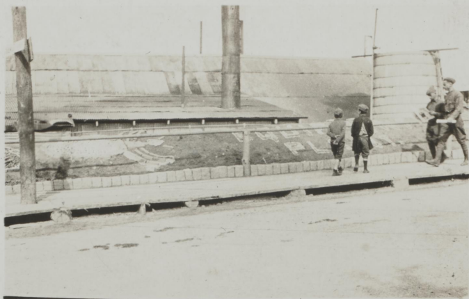
COOTIES MADE OF BRICKS - ON TERRACE IN FRONT OF PLANT
