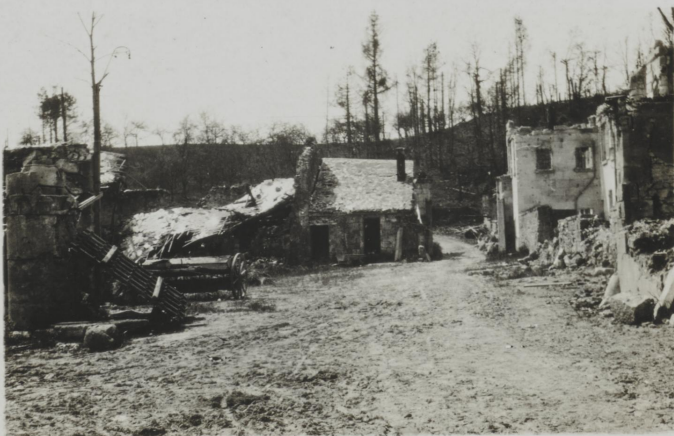
LOOKING TOWARD BARNYARD GATE FROM INSIDE
