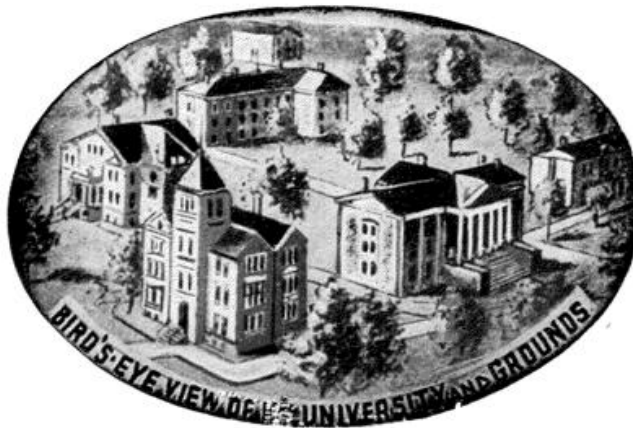
The Buildings Where Gen. Smith's College was located for 35 Years
