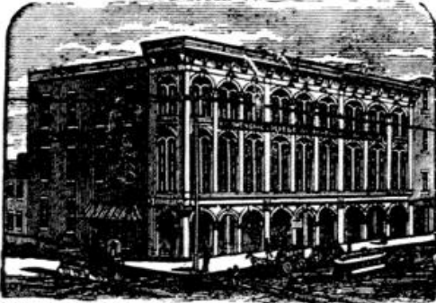
S. W. Cor. Main & Minor Sts. opp. Court House
