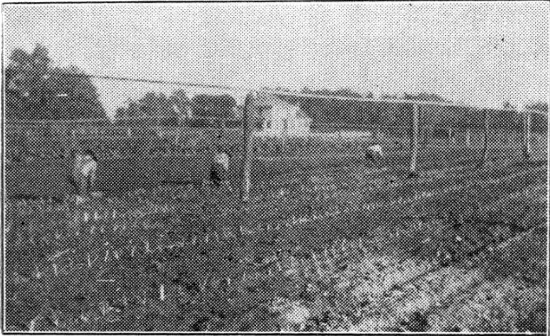
Showing Overhead Pipes Used in Irrigating Gardens.
