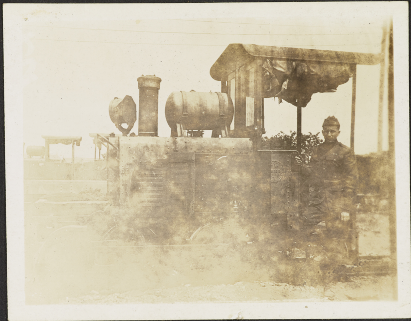
Gasoline Tractor (Locomotive) Used at extreme front - acct. silence.
