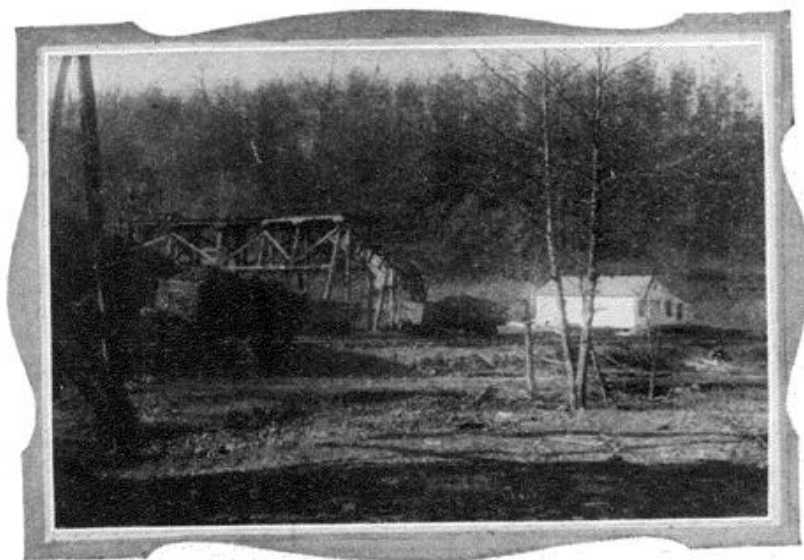
PROBABLY THE BEST CONSTRUCTED TIPPLE IN THE ENTIRE DISTRICT
