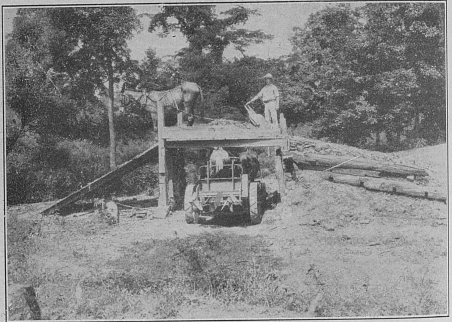
Loading marl with home-made trap-door incline. Marl spread at little or no cash outlay reduces production costs and the land improves each year.
