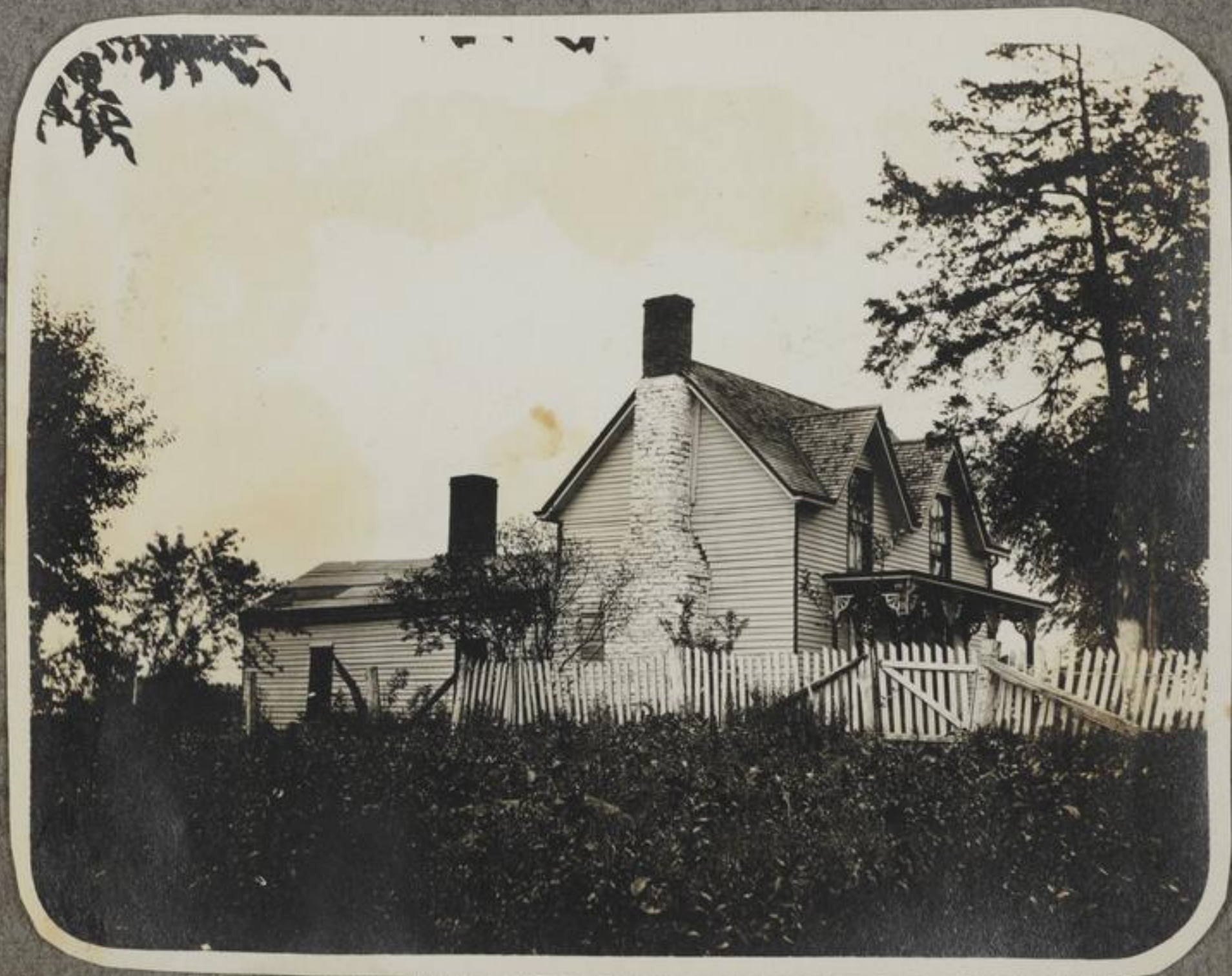
North Side the yard Fence Old Home you will notice the yard Fence we had about 2 acres is very close to the Home now in yard
