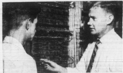
"10:45 a.m. Before any modifications can be made, it's important that I check apparatus and wiring options. That's what I'm doing here at the Remote Control Terminal equipment."
