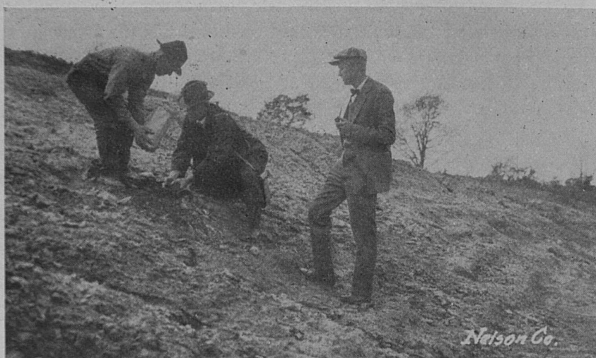
Five hundred tons of marl were removed from marl bed in the fall of 1924, only hard material being left, but it became soft during the winter and spring. This picture was taken May 1, 1925.
