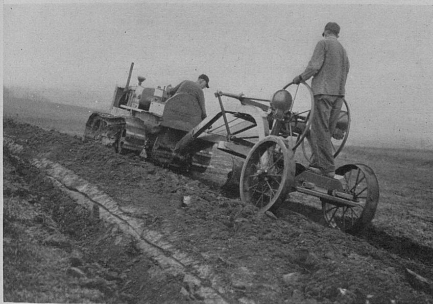
In Kentucky 10,226 acres of land were terraced and 129 farm reservoirs were constructed. This terracing unit was designed specially for Kentucky conditions.
