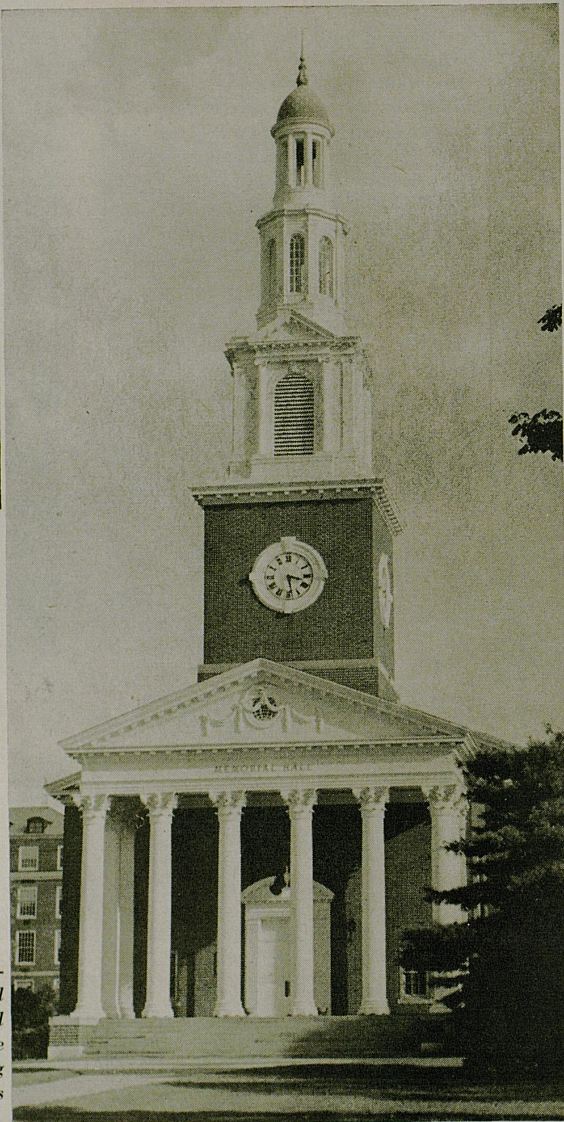
One of the lovelier buildings on the U.K. campus is Memorial Hall . . . The spire of the colonial-type building rises above one of the South's oldest universities.
