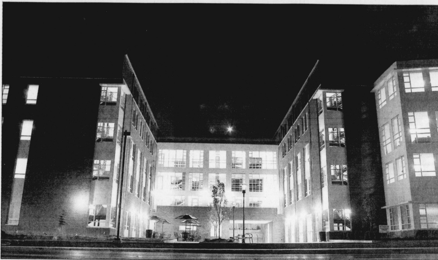
KEITH SMILEY | STAFF The new dormitory on North Campus, called "New North Hall," is one of four dorms that opened for this school year. UK also built three new dorms on South Campus. The four buildings are the first new dorms at UK since 1979, when the university unveiled the Greg Page Apartments, which are located behind Central Baptist Hospital and the arboretum off Alumni Drive.
