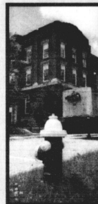
The fire hydrants outside the Administration Building were the source of problems at the beginning of the fire. DWAYN CHAMBERS | SUMMER PHOTO EDITOR
