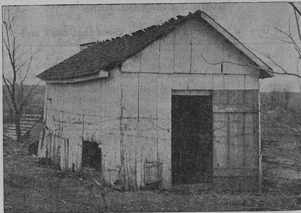
Fig. 4.—A house like this is small, dark, and poorly ventilated. Hens kept in such houses lay very few eggs in late fall and winter.
