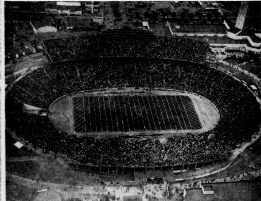
Between 60,000 and 70,000 are expected to witness the Kentucky-Southern, Methodist battle tomorrow afternoon in Dallas Cotton Bowl Stadium shown above. The huge structure has a capacity of 75,347. Oddsmakers have installed Kentucky as a 7 to 10-point favorite to whip the powerful Mustangs of Dallas.
