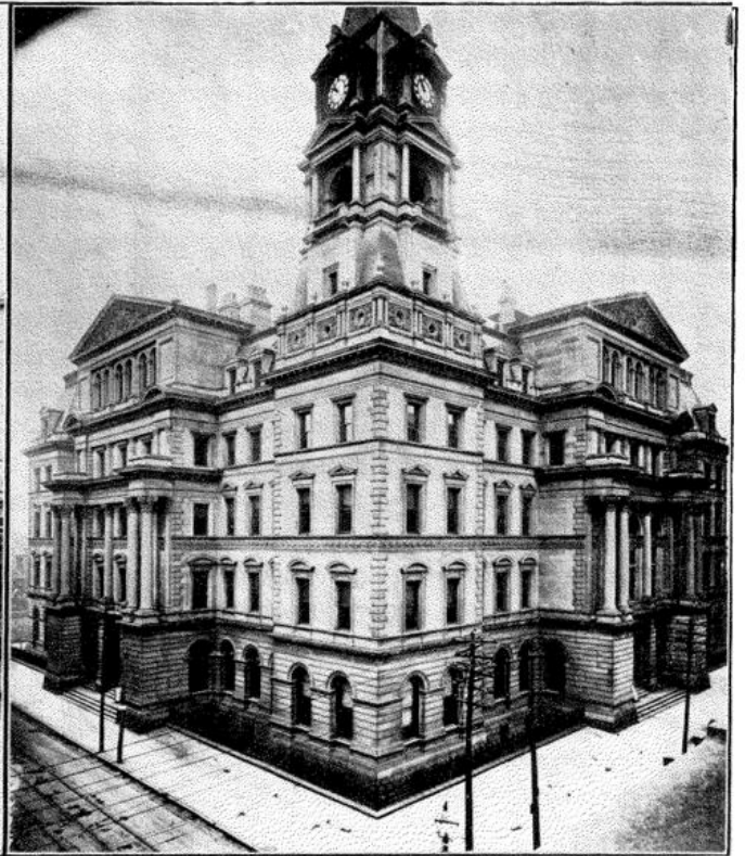
LOUISVILLE CUSTOM HOUSE
