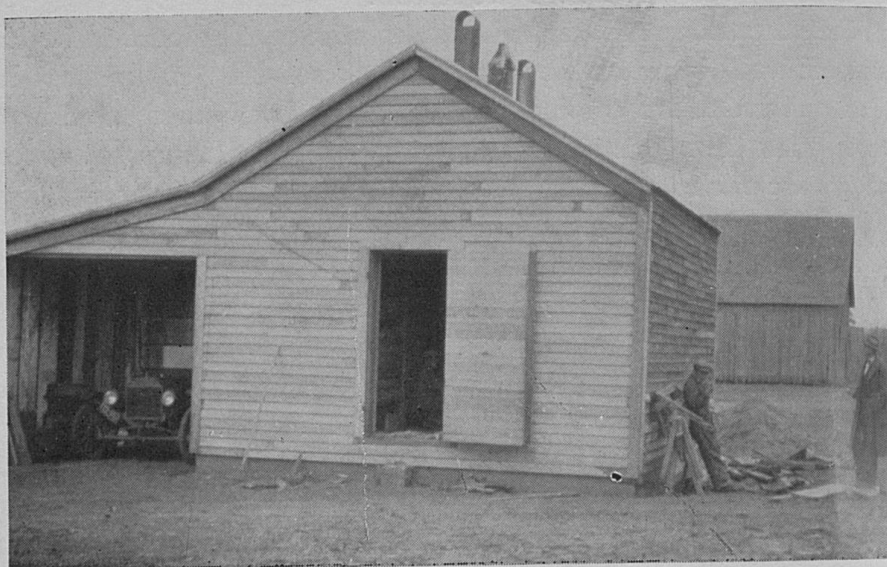
FIGURE 4. An 800-bushel sweetpotato storage house, with lean-to garage.
