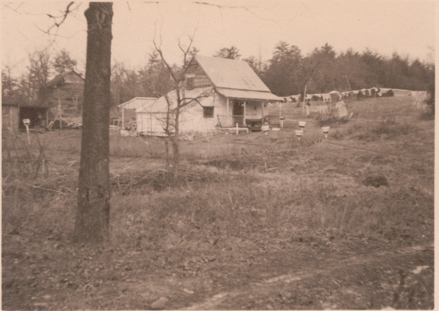
NO. 4. TYPICAL FARM OF THIS AREA
