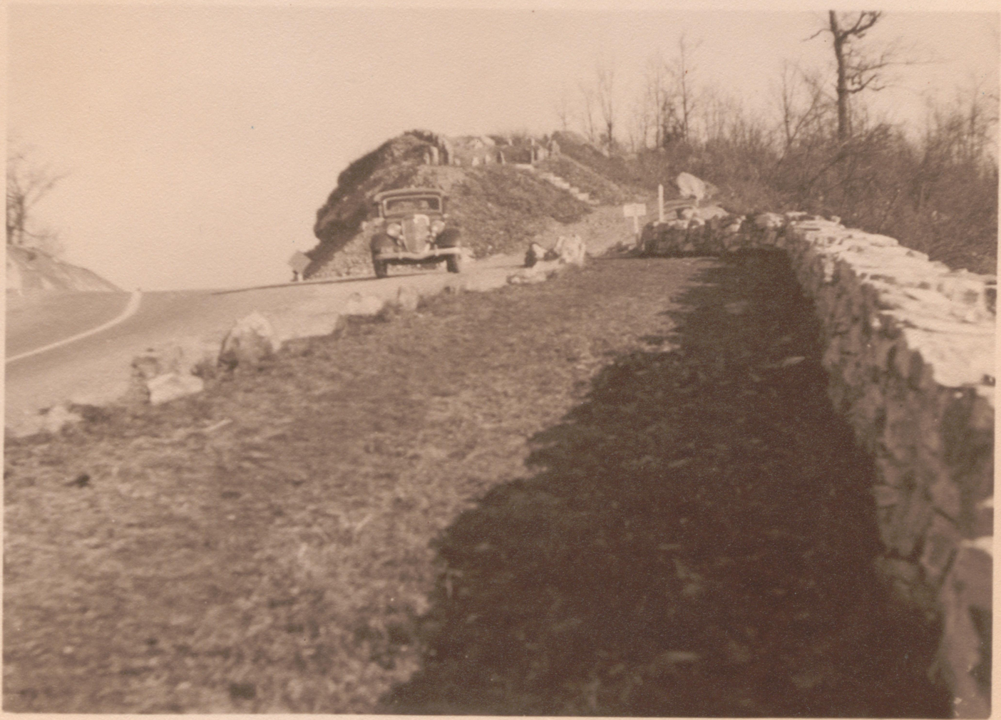
NO. 4. HIGHWAY CUT THROUGH DRAPER MOUNTAIN
